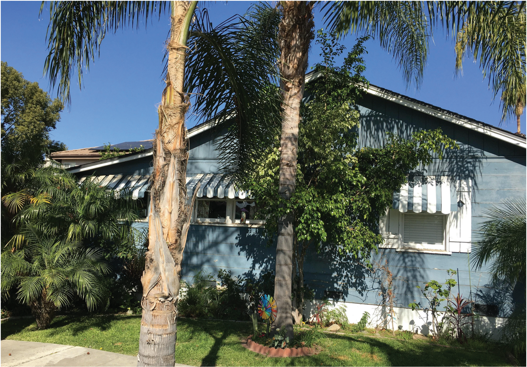
PHOTO - SOUTH SIDE - FANO STREET
