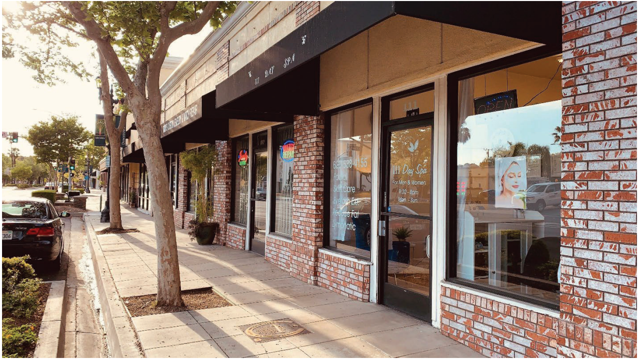
Subject Site from E. Huntington Drive
