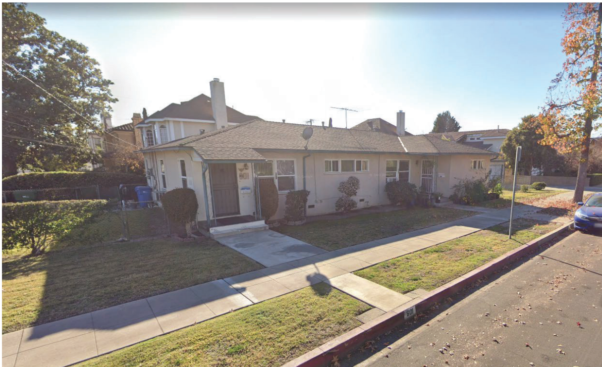
601 S. Second Avenue (south-west corner of S. Second Avenue and Fano Street, opposite the subject property)
