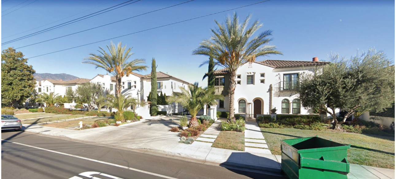
506 – 588 S. Second Avenue – Spanish style townhouse development constructed in 2015
