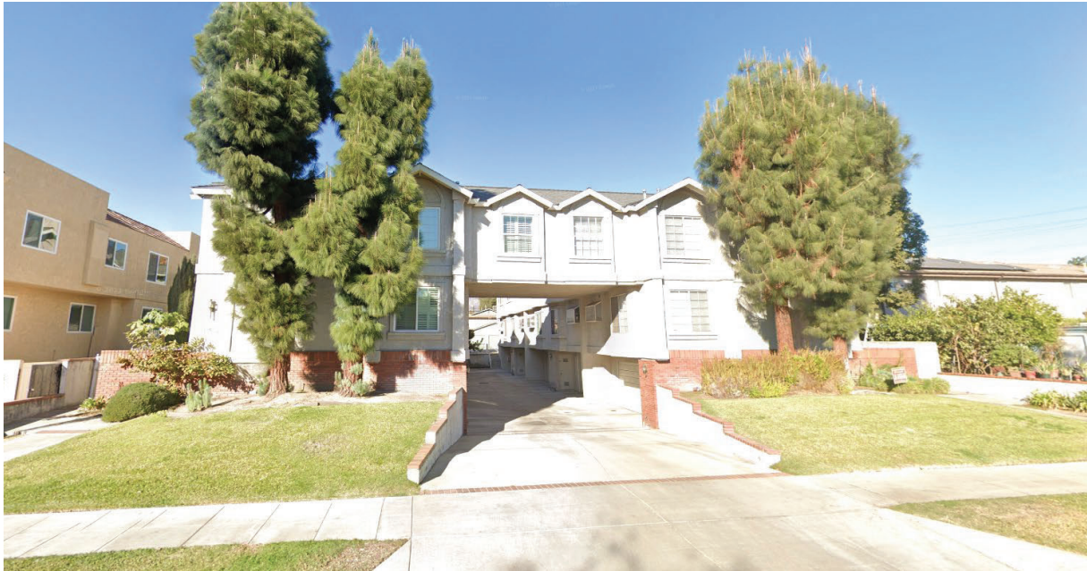
Condominiums at 153 – 157 Fano Street. Subject property is to the immediate east.
